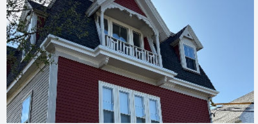
Franklin St. Fire Station - windows, boiler & spray foam replaced
