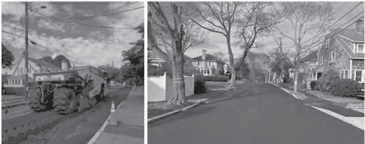
Full Depth Paving and Sidewalk Improvements West Street (left) & Mystic Road (right)
