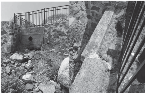
Outfall Repair Project
