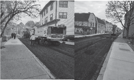
Milling and Sidewalk Rehabilitation State Street
