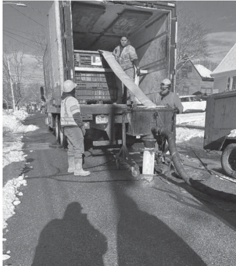
Figure 3 -Trenchless Technology Lining of Sewer Mains
