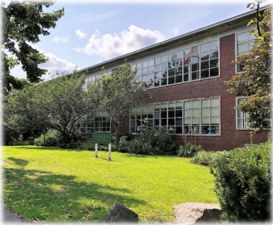
Entrance/front of the former Coffin School (Image Source: Wicked Local )
