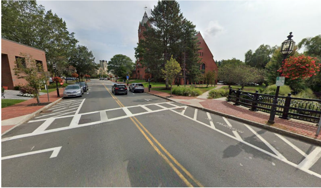
Figure 25: Daylighting at a trail crossing in Winchester, MA
