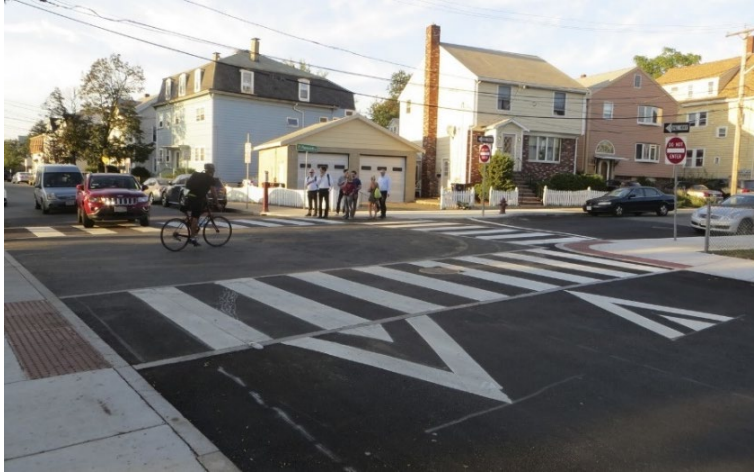
Figure 38: Raised intersection in Everett, MA
