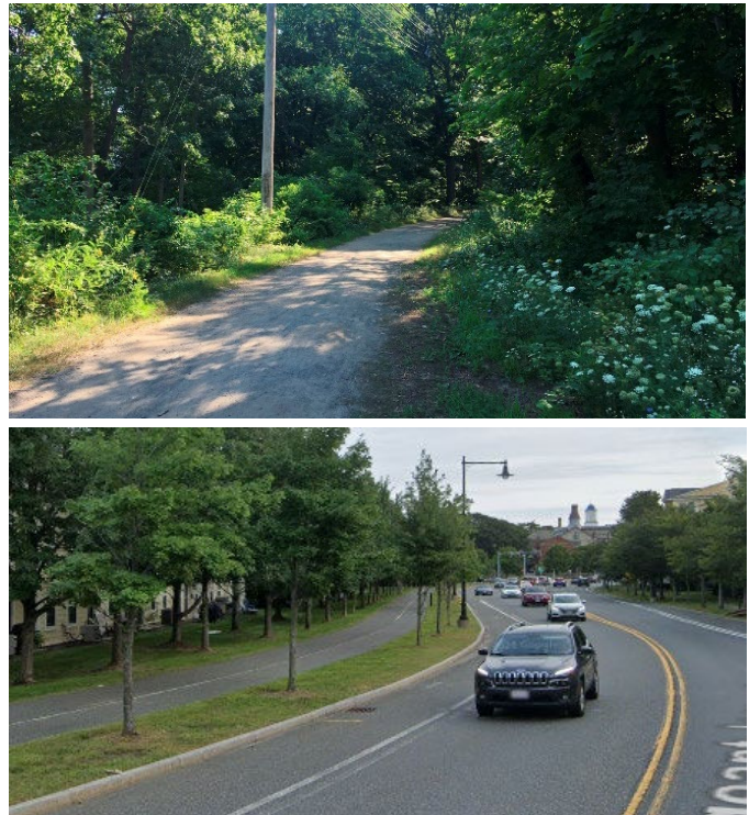
Figure 18: Marblehead Rail Trail (top) and a shared use path along a roadway in Salem, MA (bottom)
