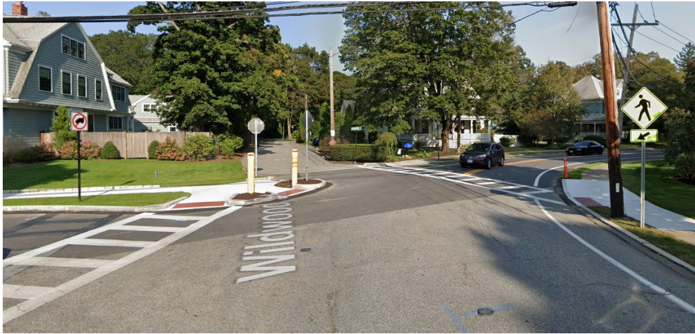
Figure 36: Irregular Intersection Geometry at Winchester, MA
