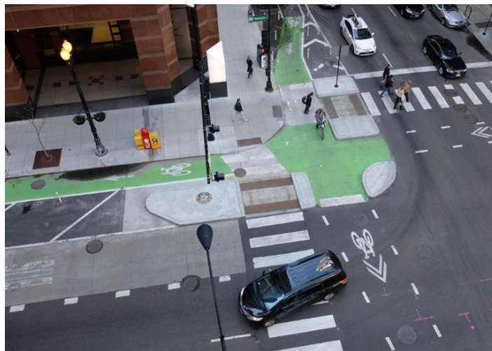
Figure 37: Protected Intersection in Oakland, CA
