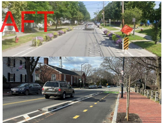
Figure 20: Quick-build separated bike lane with planters Burlington, VT (top), and two-way separated bike lane with concrete parking stops in Cambridge, MA (bottom)
