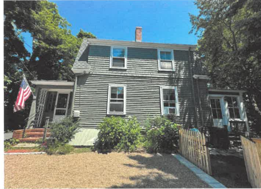
FRONT FACADE. VIEW FROM DRIVEWAY, VISIBLE FROM STREET
