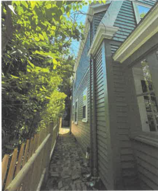
SIDE ALLEY. VIEW FROM HARDING LANE STREET
