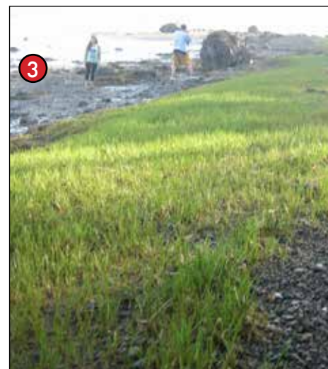
Coconut fiber mats were used to establish marsh grasses.
