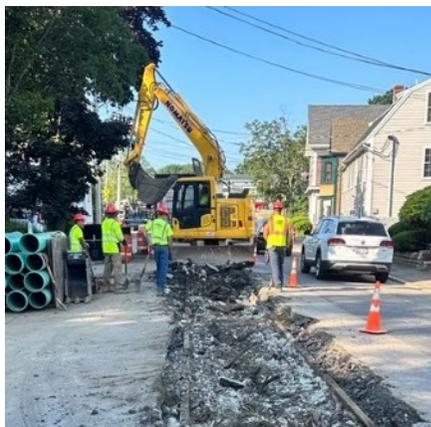
**Rail Tracks found under Bessom Street Storm Sewer System Extension Project**
