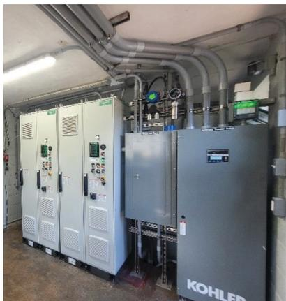
Figure 2 - New VFD's and electrical panel in Green Street Pumping
