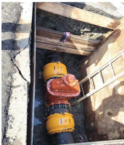
*Figure 21 – Blowoff replacement on 16” transmission line in Swampscott*
