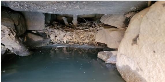
**Blockage cleared during storm sewer maintenance**
